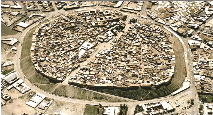
Aerial view of Erbil Citadel
